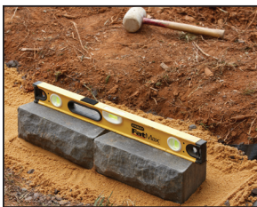
4. Lay and level blocks
