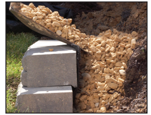
5. Add drainage aggregate
