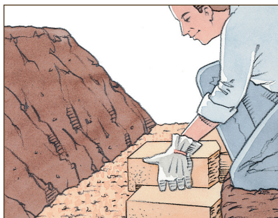
Diagram 3—Next-Course Construction
